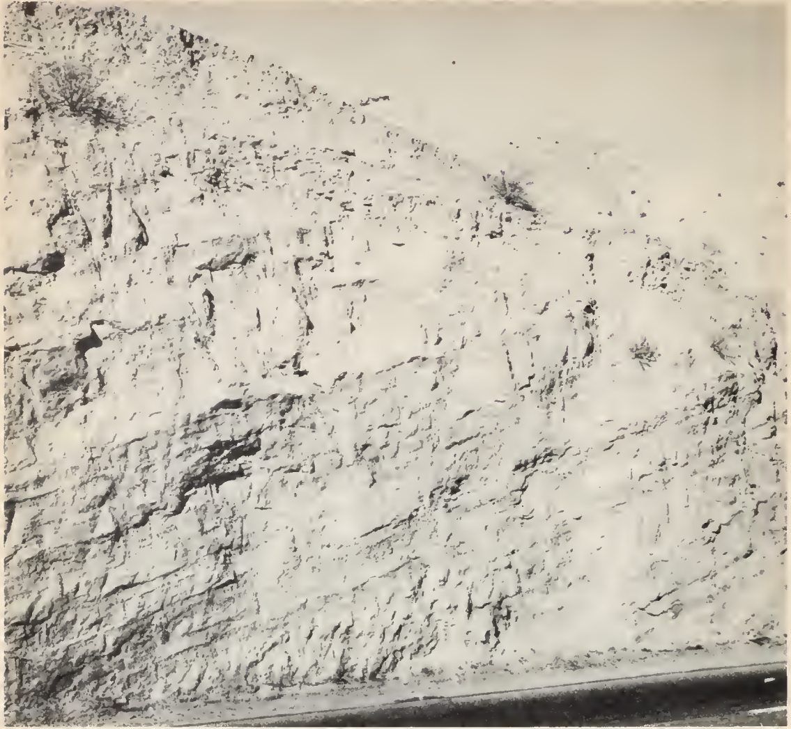
FIGURE 19. Walker beds exposed in cut on Highway U. S. 466, one mile west of Ilmon.
